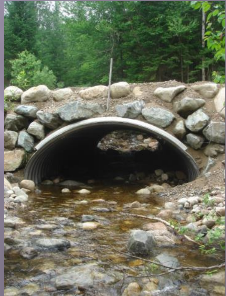
Post-replacement – looking upstream July 2013
