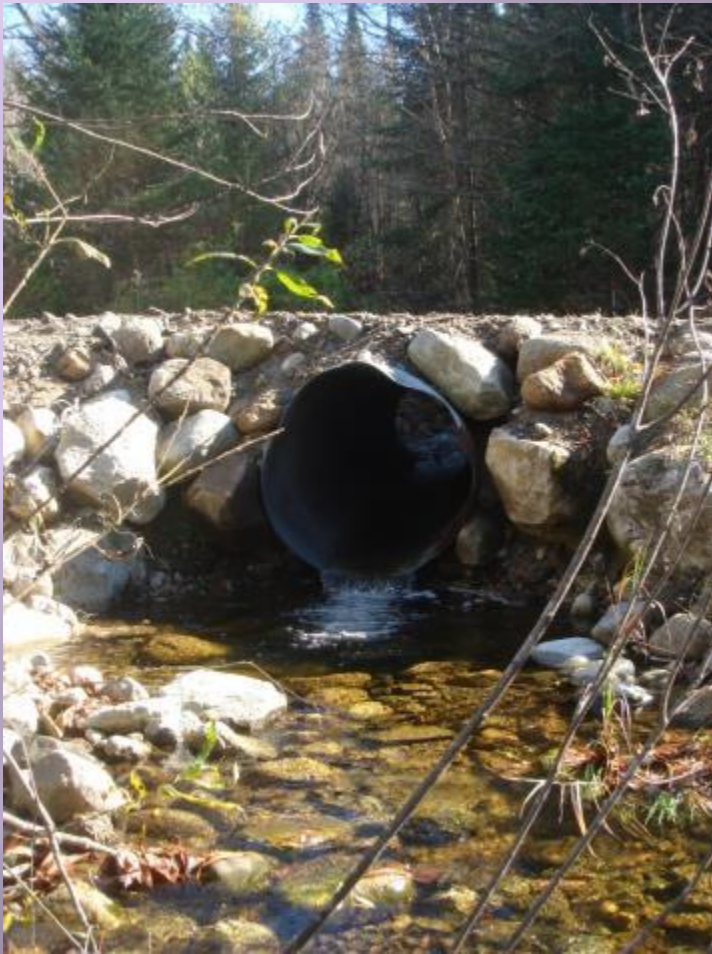
Pre-replacement – looking upstream October
