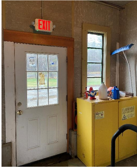
Figure 6-9: Entrance Bay Main Entrance Door
