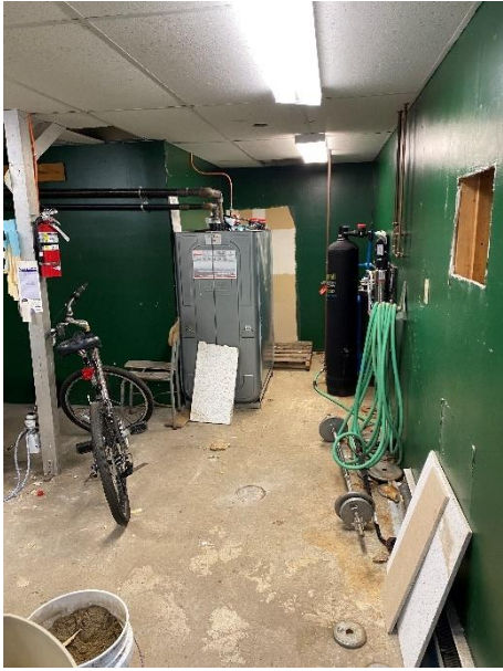
Figure 6-26: Mechanical Room cut outs in wall
