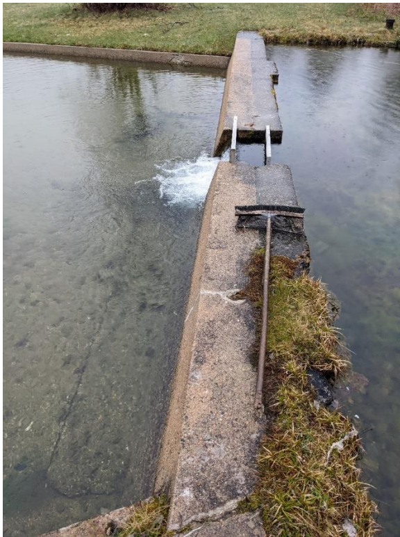
Figure 4-5: Pump 1 Reservoir Dam
