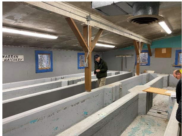
Figure 5-5: Linear Tanks in Rear Addition
