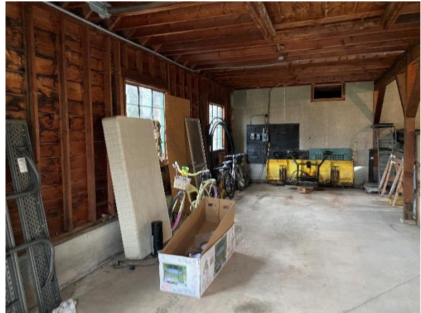
Figure 6-6: Garage Bay Rear Wall
