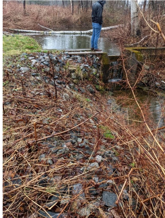
Figure 4-9: Dam/Impoundment of Pump 3 Reservoir (Screen Box in left background)
