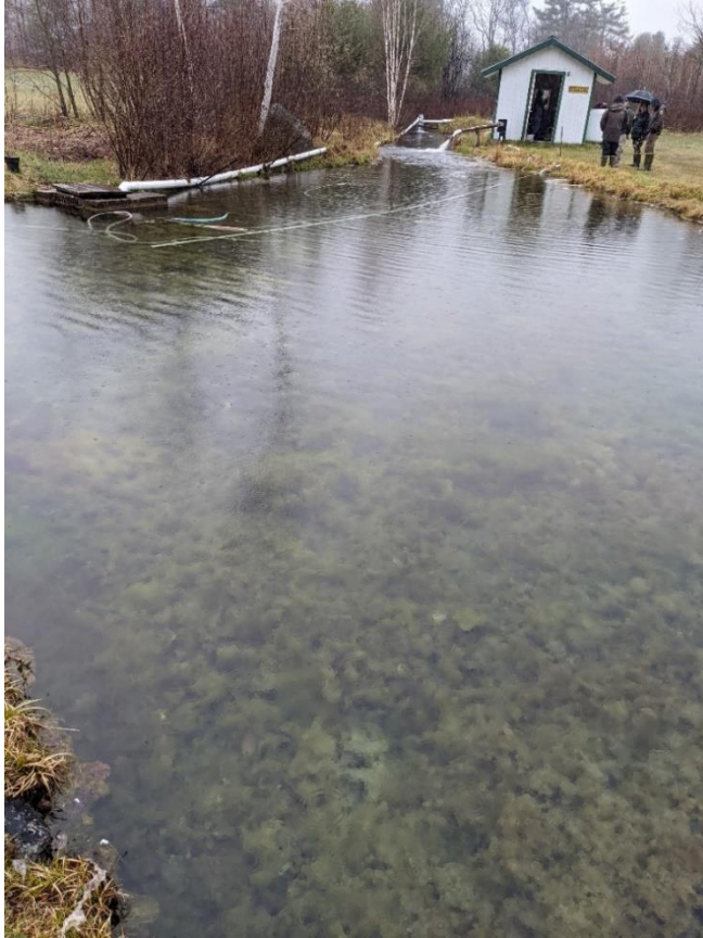
Figure 4-1: Well/Pump House #1 and Spring Reservoir
