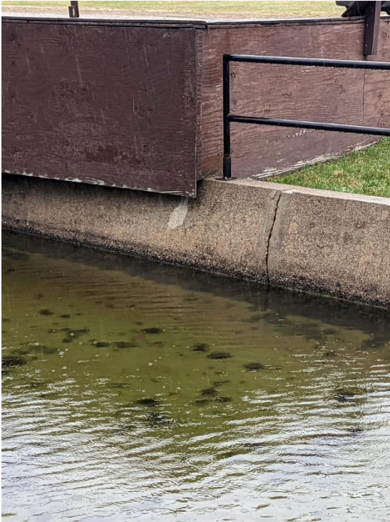
Figure 5-38: Viewing Deck at Big Show Pond
