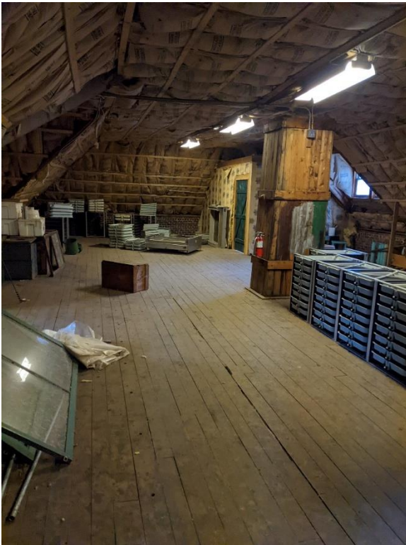
Figure 5-7: Hatch House Building Attic Area
