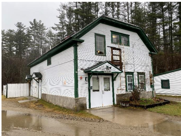
Figure 6-20: Visitor Center North Side Facade
