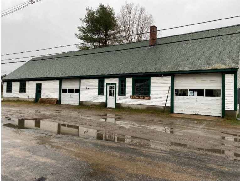
Figure 6-4: Warehouse Building Front Facade
