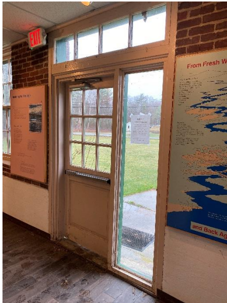
Figure 5-12: Front door from interior
