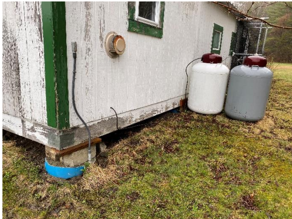
Figure 6-18: Southeast Corner of Feed Storage and Pole Shed
