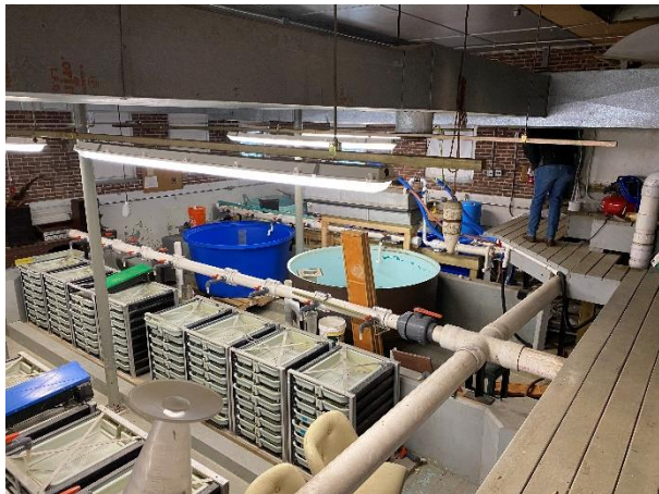
Figure 5-20: Tank Room view from walkway
