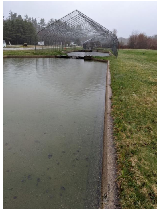
Figure 5-29: Predator Protection Structures at Middle Reservoir Pond
