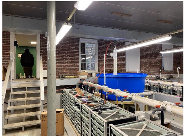
Figure 5-21: Tank Room view of main stairs
