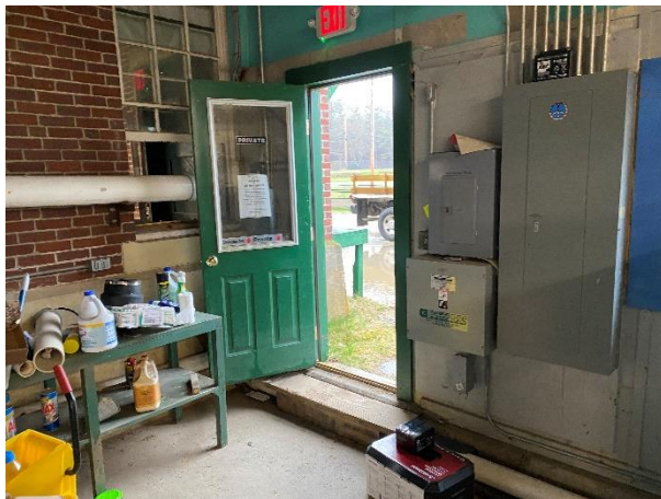
Figure 5-16: Rear Addition Door Interior
