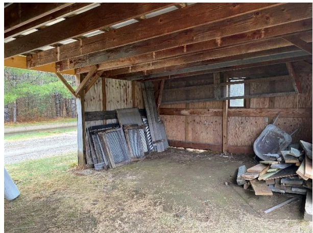
Figure 6-16: Storage Shed Interior
