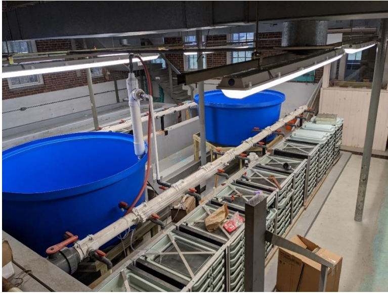
Figure 5-9: Hatch House Production/Incubation Area
