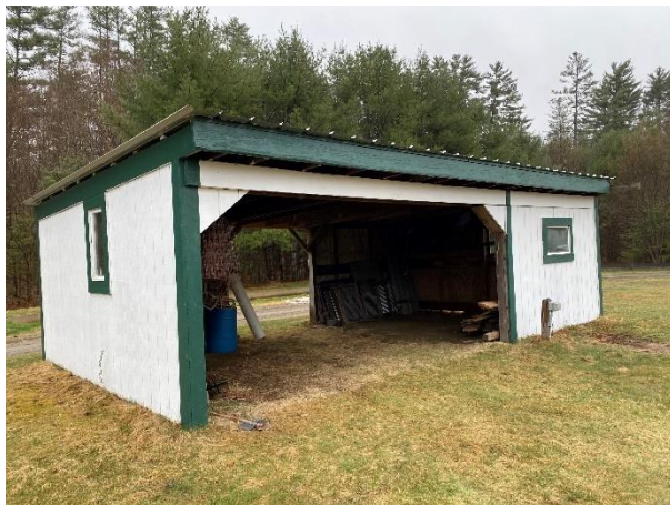
Figure 6-15: Storage Shed Front View
