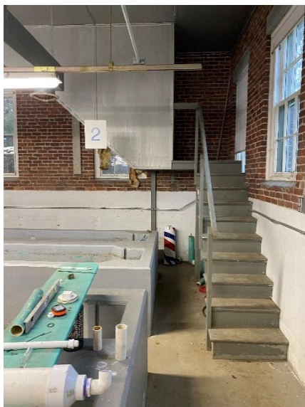
Figure 5-22: Access stairs to attic
