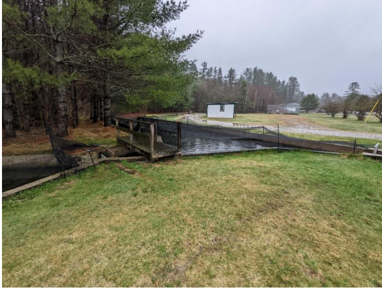
Figure 5-40: Storage Shed in Center, Clarifiers in Background, Below Bridge Pond in Foreground.
