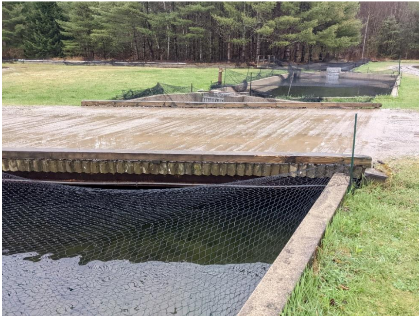
Figure 5-32: Bridge Pond Raceway and Timber Bridge
