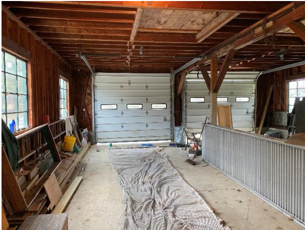
Figure 6-5: Garage Bay Overhead Doors
