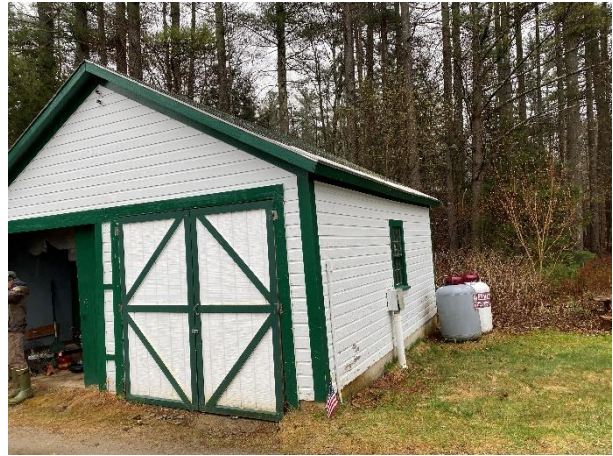
Figure 6-3: West Facade Electrical Connection and Propane Tanks
