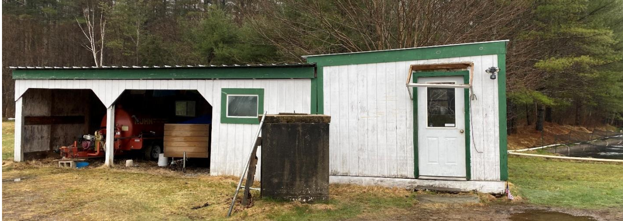
Figure 6-17: Feed Storage and Pole Shed Front (West) Facade
