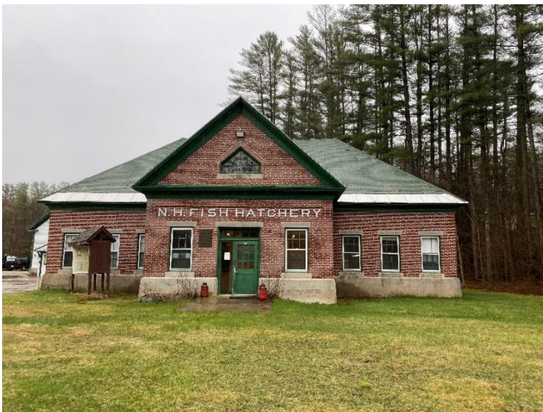
Figure 5-1: Hatch House Front (West) Facade
