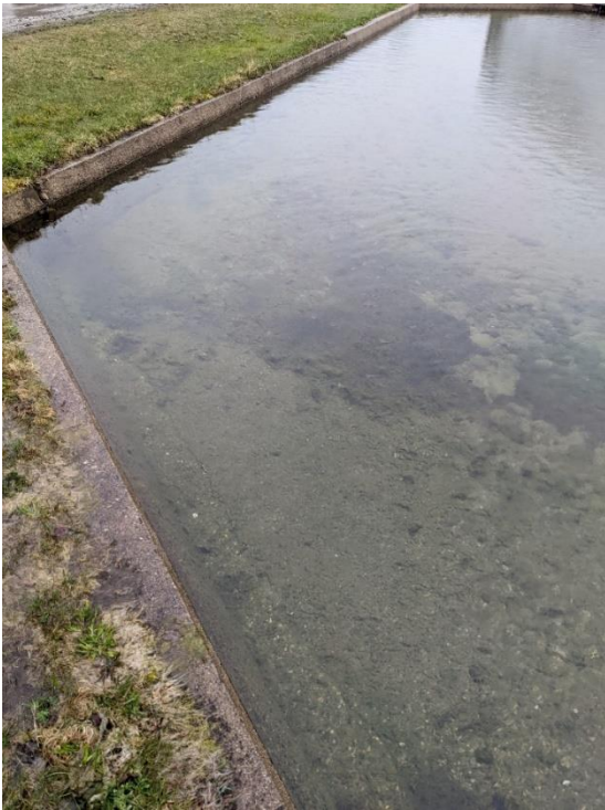
Figure 5-28: Walls at Upper Reservoir Pond
