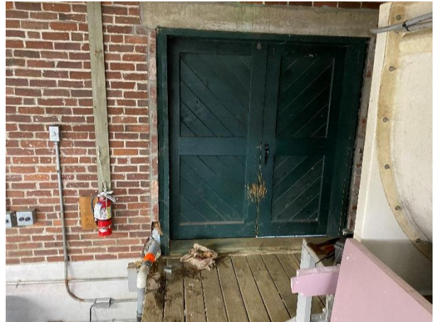
Figure 5-15: Loading Dock Door from Inside
