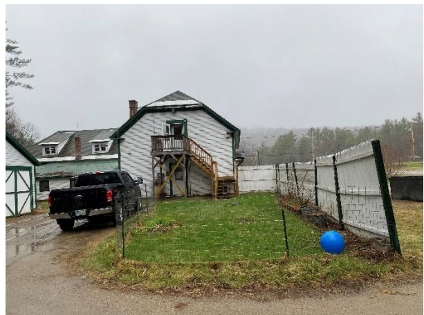
Figure 6-21: Rear View & Exterior Stair Access to Upper Level
