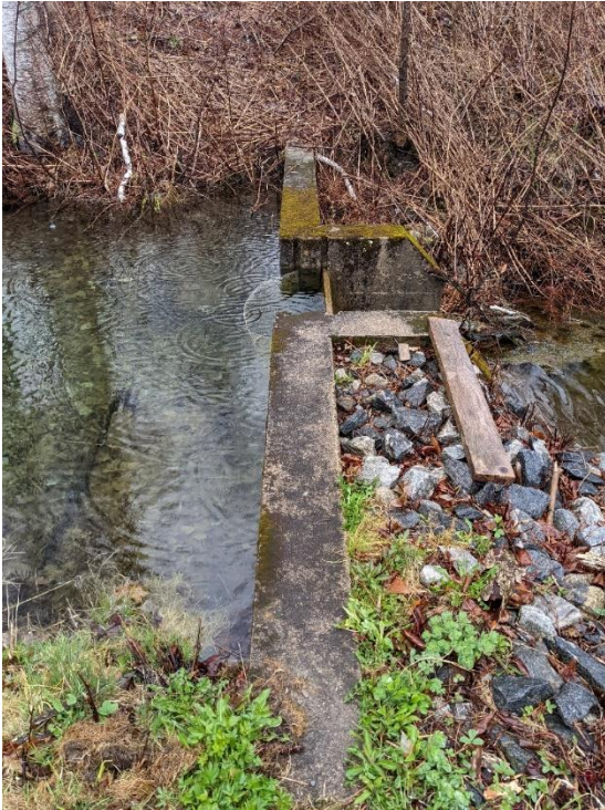
Figure 4-8: Impoundment/Dam of Pump 3 Reservoir
