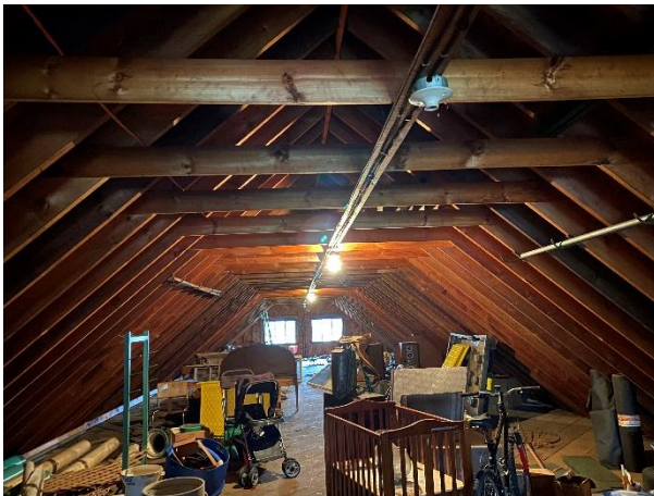
Figure 6-13: Attic Space Storage Area
