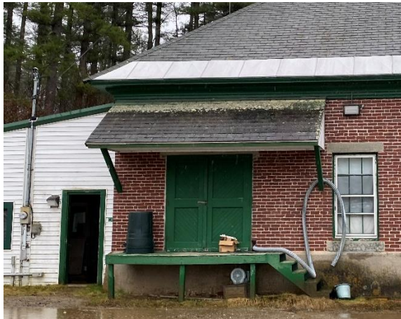
Figure 5-14: Side Loading Dock Door
