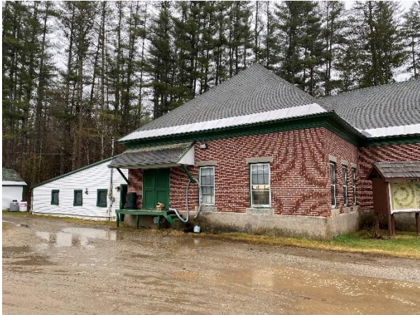
Figure 5-2: Hatch House North Facade
