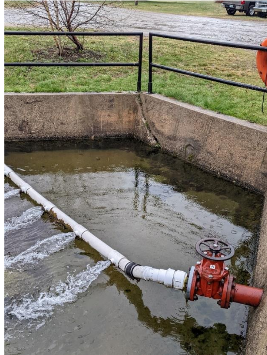
Figure 5-39: Typical Wall Cracking at Show Pond
