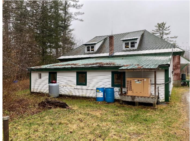
Figure 5-3: Hatch House Rear Facade
