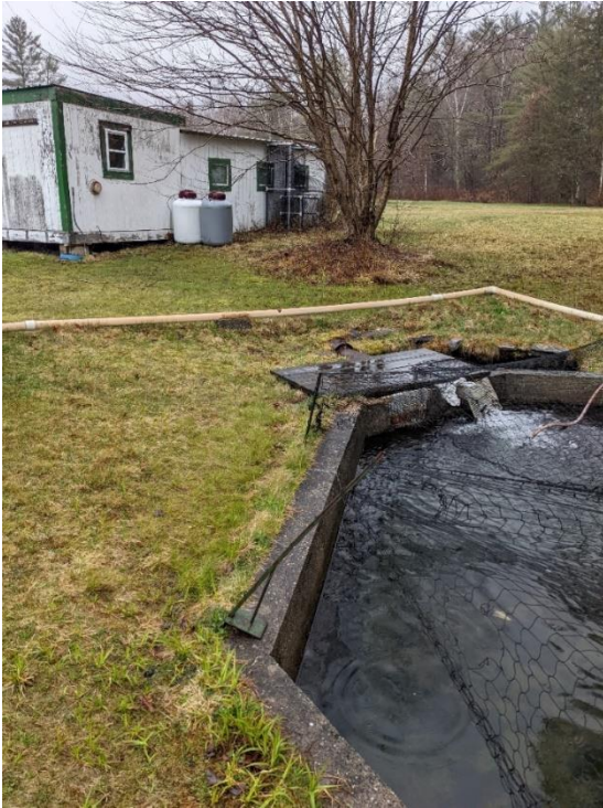
Figure 5-33: Inlet Area of Spring Pond
