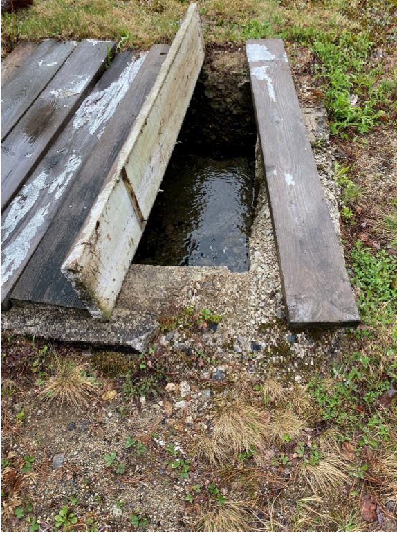
Figure 4-6 Low Producer Spring Headbox
