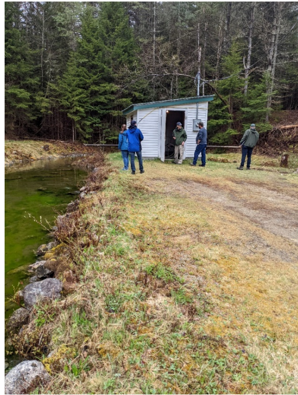
Figure 4-8: Well / Pump Building between Left and Right Springs
