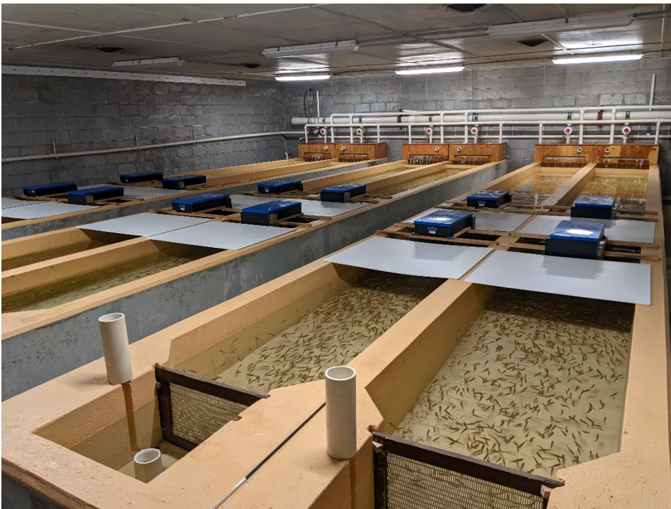
Figure 5-2: Indoor Raceways 6-11 with Fish Feeders (blue belt feeders)
