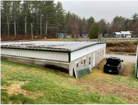
Figure 5-7: Hatch House – Low Slope Roof
