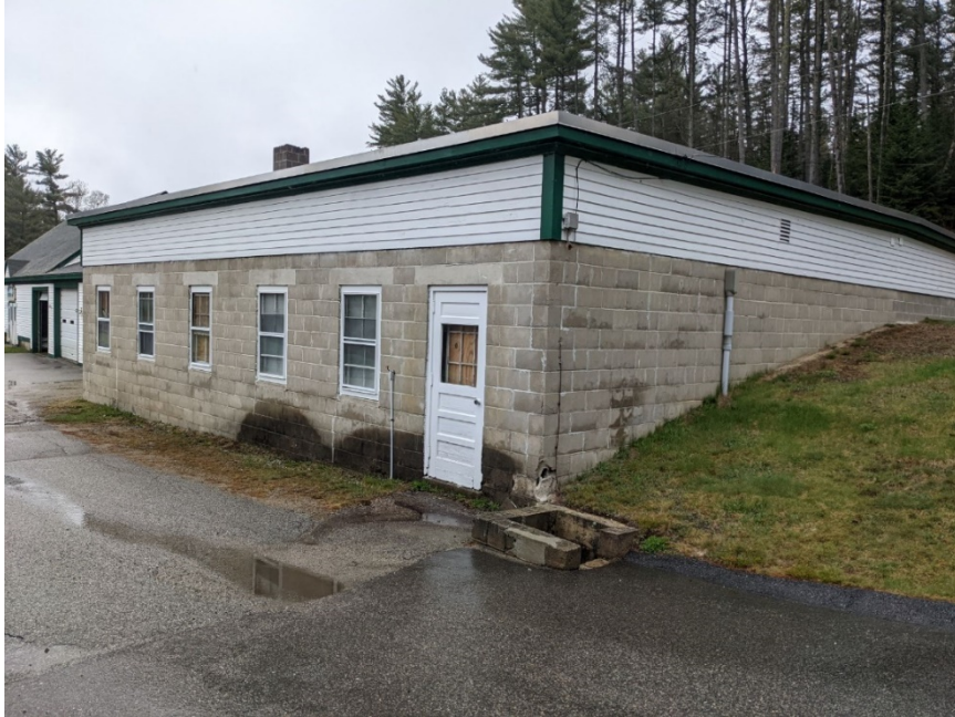
Figure 5-4: Front Face of Hatchery Building
