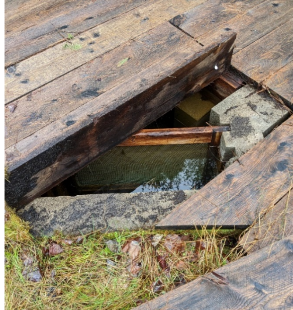
Figure 4-2: Screening Structures Below Wooden Cover of Covered Spring
