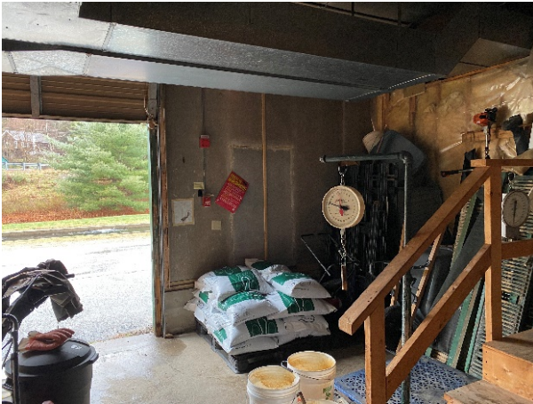
Figure 7-3: Feed Storage Bay Interior View
