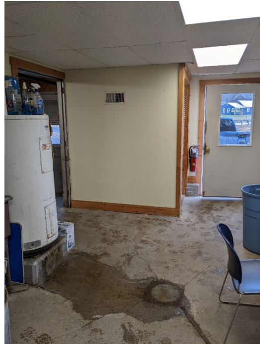
Figure 7-10: First Level of Garage/Office Building
