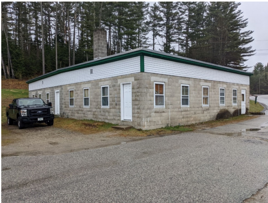
Figure 5-5: Hatchery Building North and West Faces
