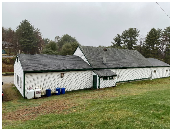
Figure 7-2: Visitor's Center Garages Rear View
