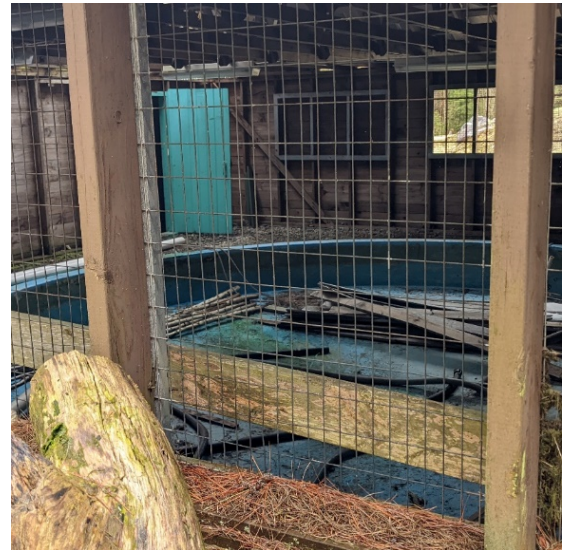
Figure 6-2: Typical Interior Tank in Broodstock Building (Abandoned)
