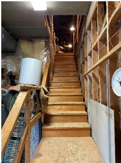
Figure 7-5: Stairs to Storage Attic
