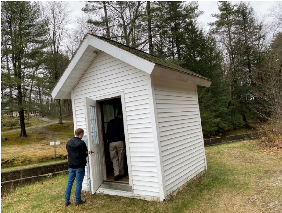
Figure 1-17: Outfall Sampling Shed
