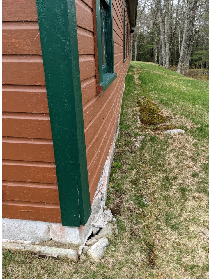
Figure 1-19: Feed Storage Building
