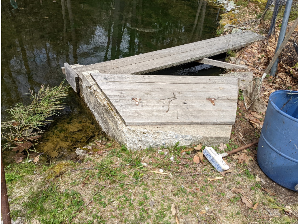
Figure 1-14: Woods Pond Outlet Box
