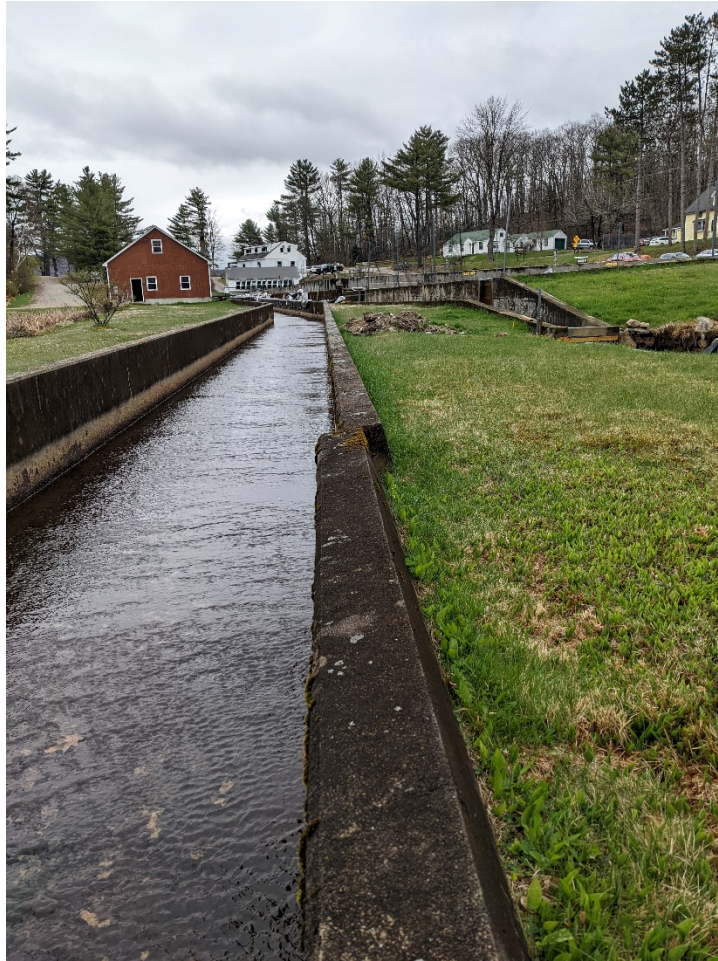
Figure 1-12: Lake Overflow Channel
