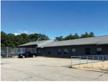
Building two at NHFG headquarters
