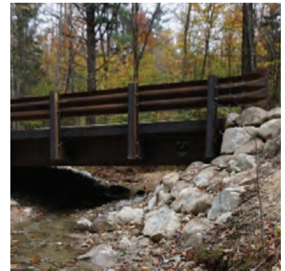
Ryan Brook bridge project in Campton
