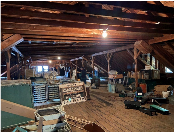
Figure 5-24: Attic overall view
