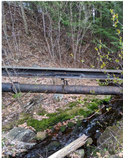
Figure 4-13: Lower crossing of Dickerman Creek for C-Series inlet pipe
