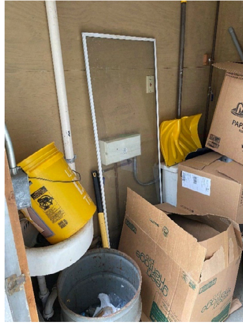
Figure 5-16: Bathroom used for storage
