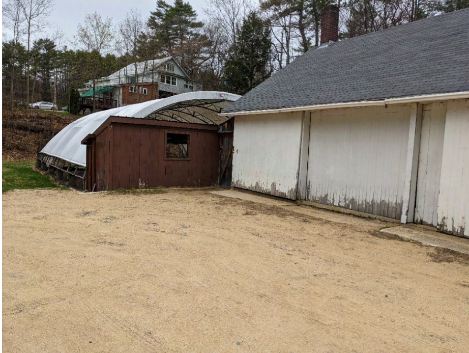
Figure 5-30: Metal Framed Plastic Cover over 4 of the 10 Raceways in Raceway A-3
