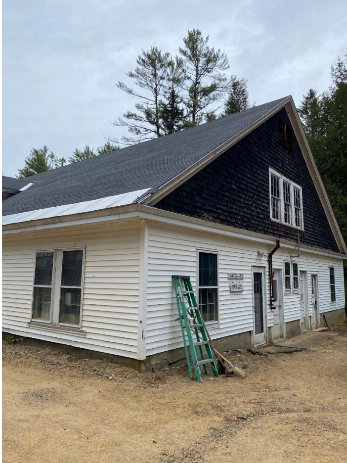
Figure 5-10: Hatch House - South (Front) Elevation
