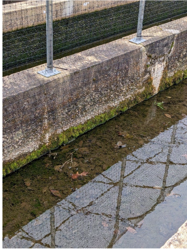
Figure 5-45: Original, unrepaired concrete surfaces at C-Series
