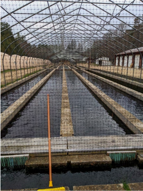
Figure 5-41: C-Series looking downstream
