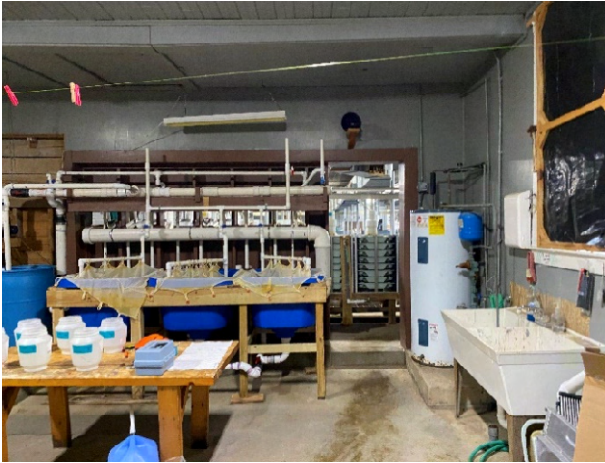
Figure 5-26: Lab Space looking south into Production Area
