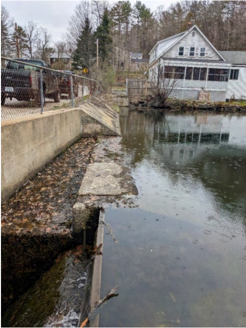
Figure 4-10: Dam at Dickerman Pond
