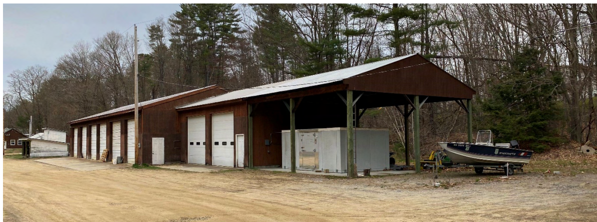
Figure 7-10: Garage - Overall View
