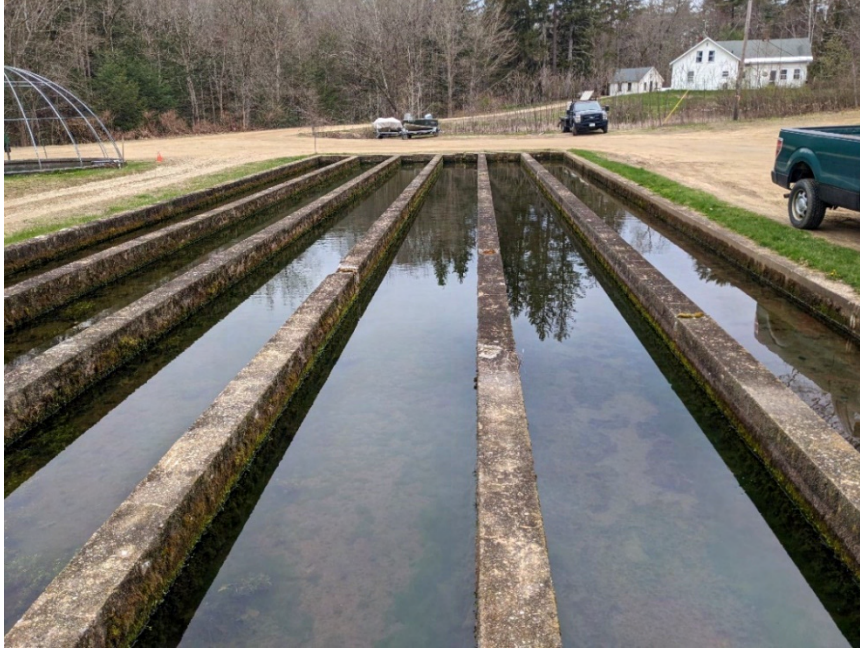
Figure 5-43: Westmost set of C-Series raceways used for treatment
