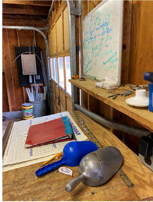
Figure 7-8: View of gaps in overhead door
