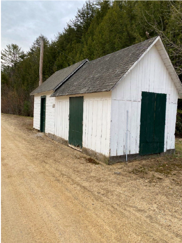
Figure 7-23: Tool Shed (Front)
