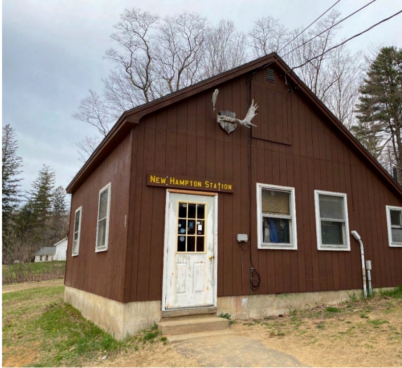
Figure 7-25: Utility Shed (C Station Office) East Façade
