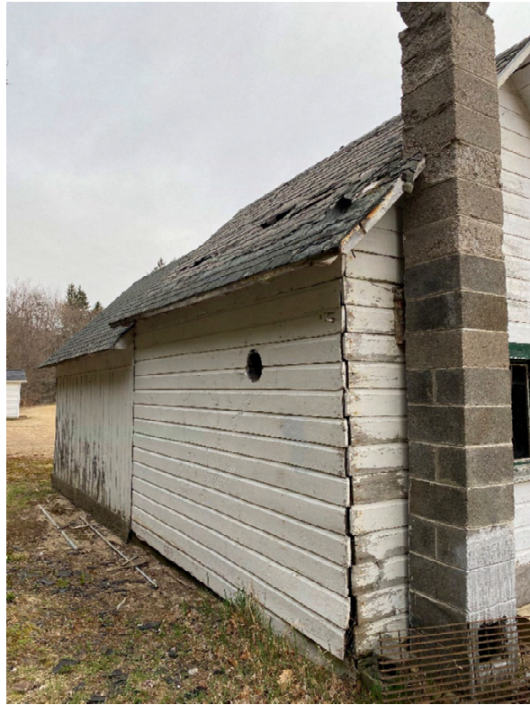
Figure 7-24: Tool Shed (Rear)
