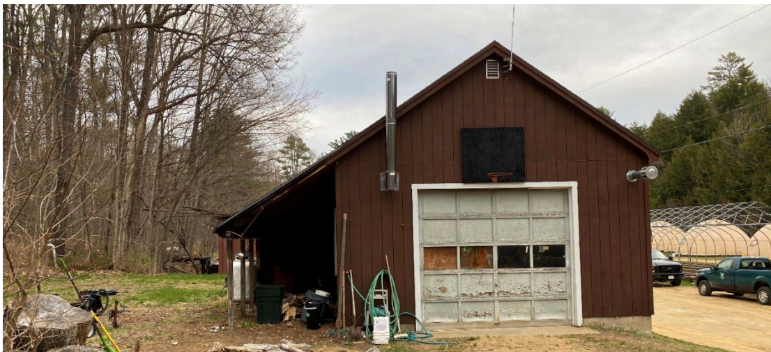
Figure 7-26: Utility Shed - West Façade
