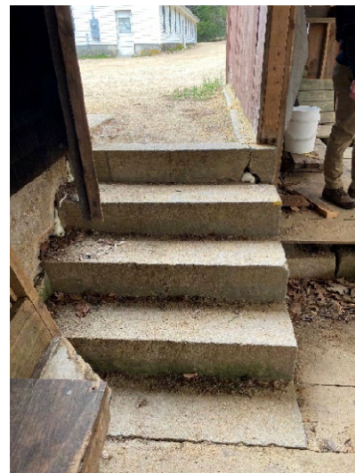
Figure 5-35: Raceway A-3 Covered Entrance Stairs
