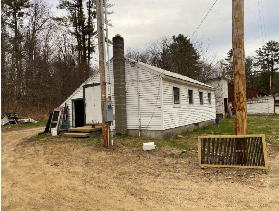
Figure 7-20: Woodworking Shed exterior view looking east
