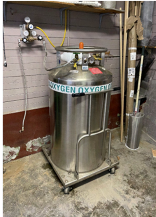
Figure 5-5: Liquid Oxygen (LOX) Tank
