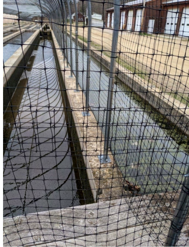
Figure 5-42: Northerly raceway at C-Series not protected by frame/netting (typical)
