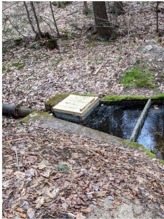
Figure 4-9: Head Box at Minor Water Source Across RT 132
