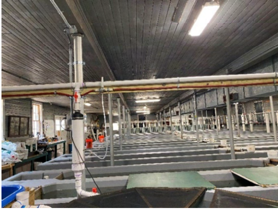
Figure 5-2: Hatch House Main Production Rearing Area
