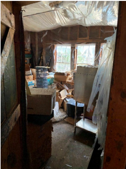
Figure 5-22: Attic Storage Room
