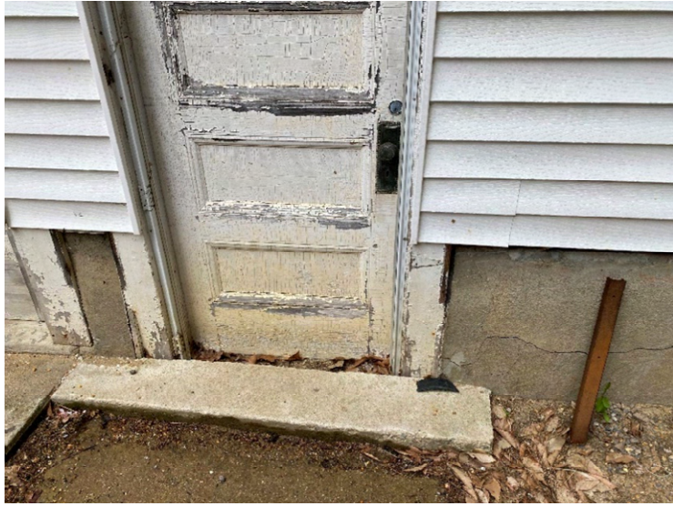
Figure 5-12: Door to Storage Room
