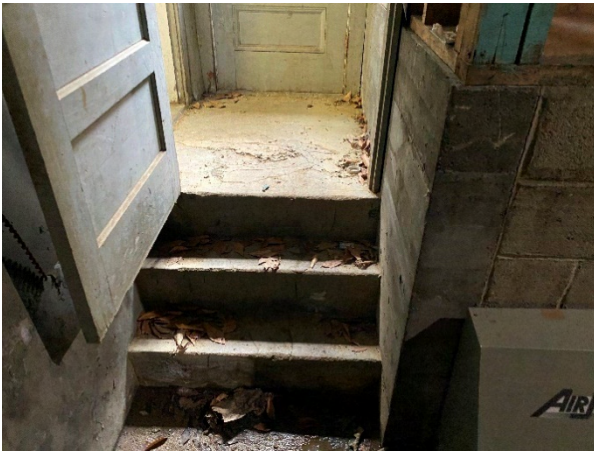
Figure 5-18: Stairs and Vestibule to Mechanical Room
