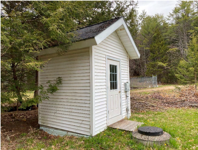
Figure 6-1: Sampling Shed at Raceway A-3
