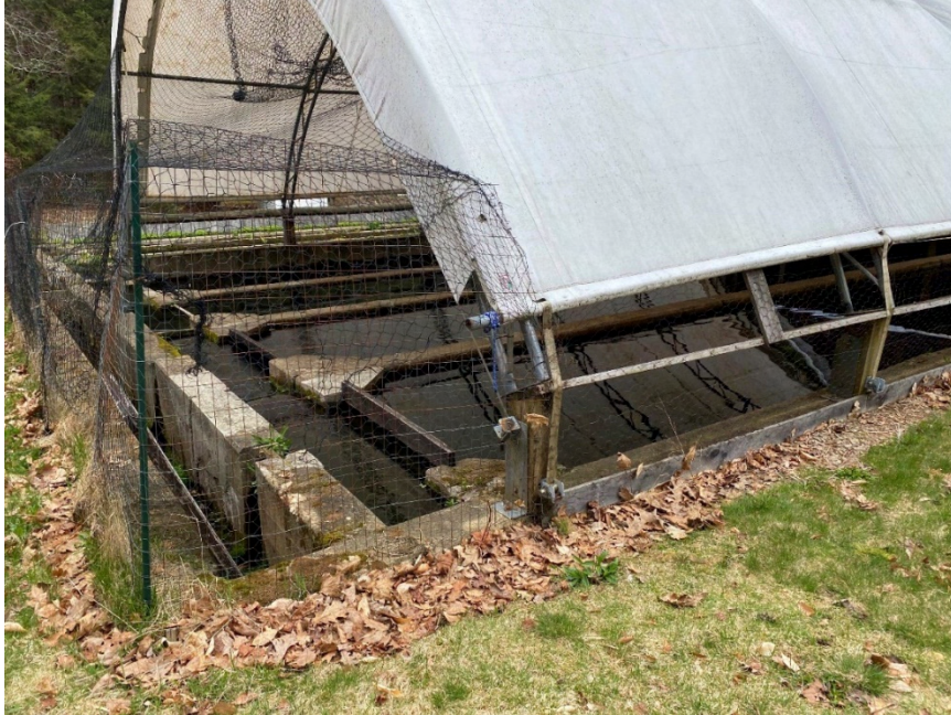
Figure 5-33: Raceway A-3 Broodstock Covering
