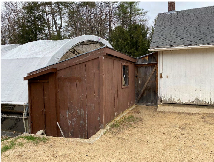
Figure 5-34: Raceway A-3 Covered Entrance Shed Structure
