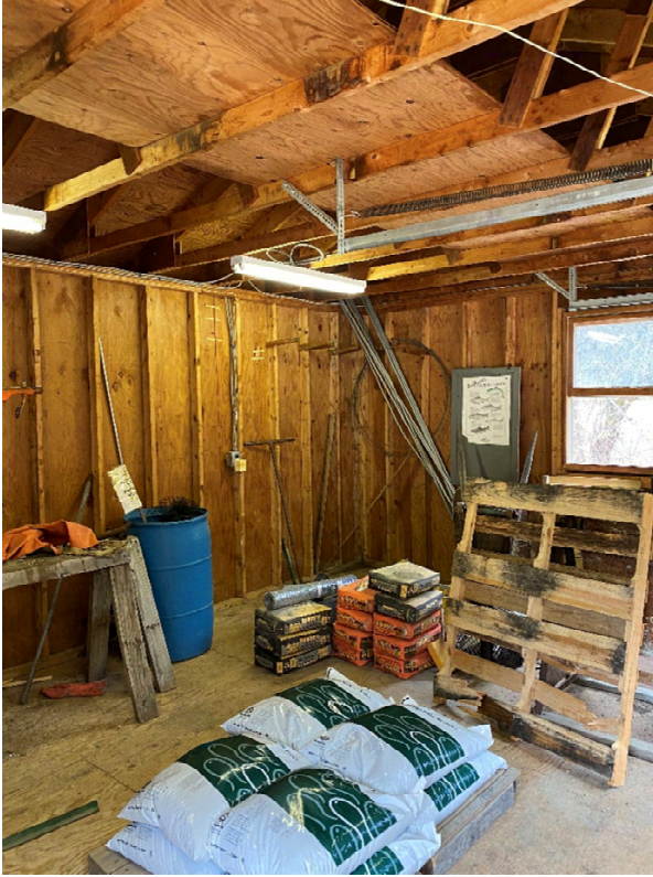
Figure 7-7: Interior View of Feed Shop
