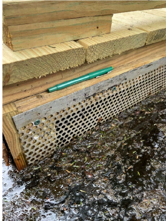
Figure 4-7: Wood Framed Inlet Screen at Minor Spring
