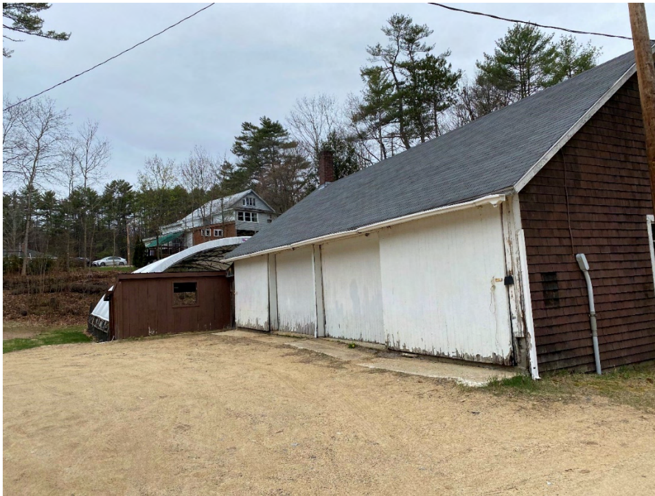
Figure 7-1: Upper Garage Front (South) Façade
