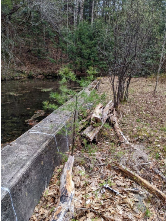
Figure 4-3: Sealed Surface Cracks in Spring Pool
