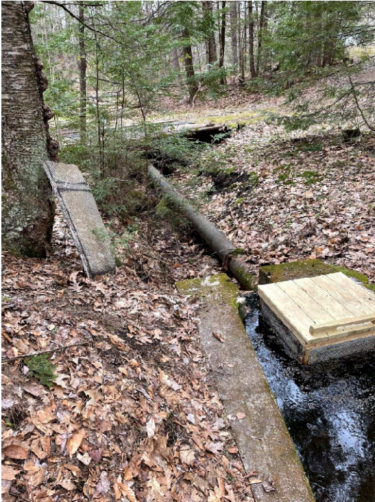
Figure 4-6: Minor Spring Concrete Headbox
