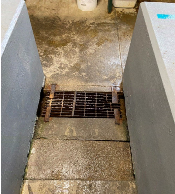
Figure 5-8: Drainage Channels
