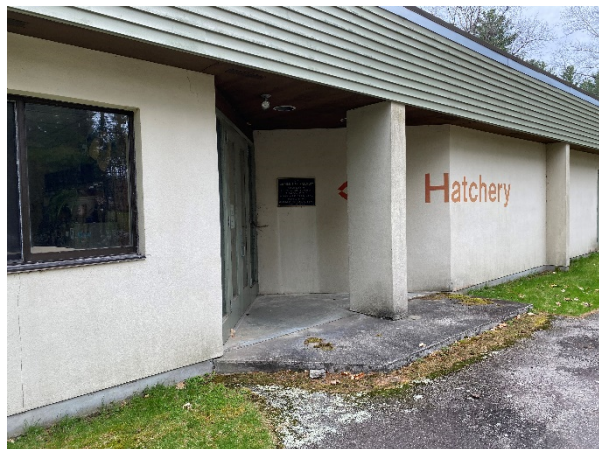
Figure 3-7: Main Public Entrance
