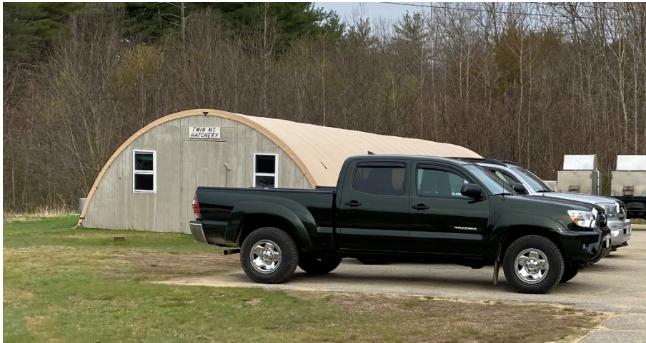
Figure 5-25: Twin Mountain Hatchery Hut
