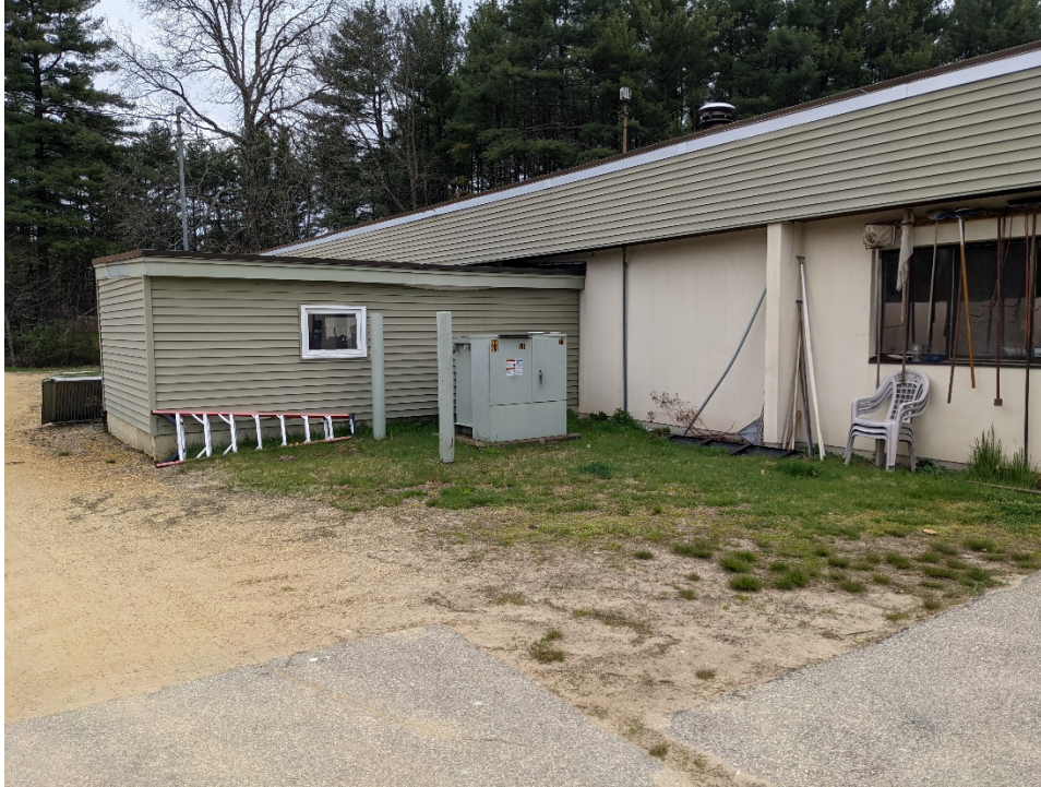
Figure 5-4: Rear Facade of Hatch House and Addition
