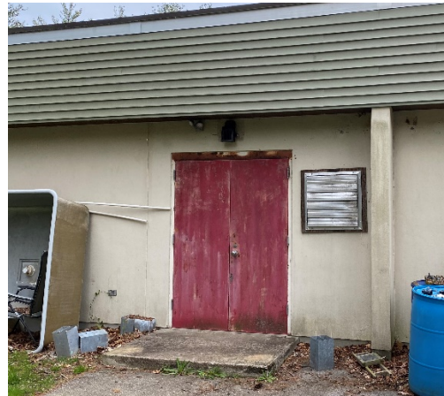
Figure 5-9: Doors to Tank Room
