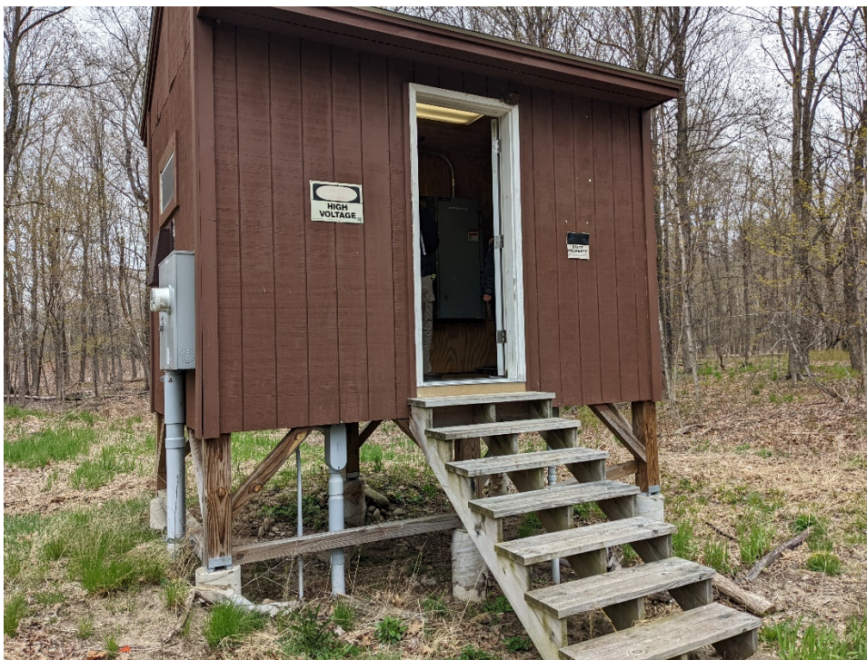
Figure 4-4: Newer River Well (No. 4) Structure
