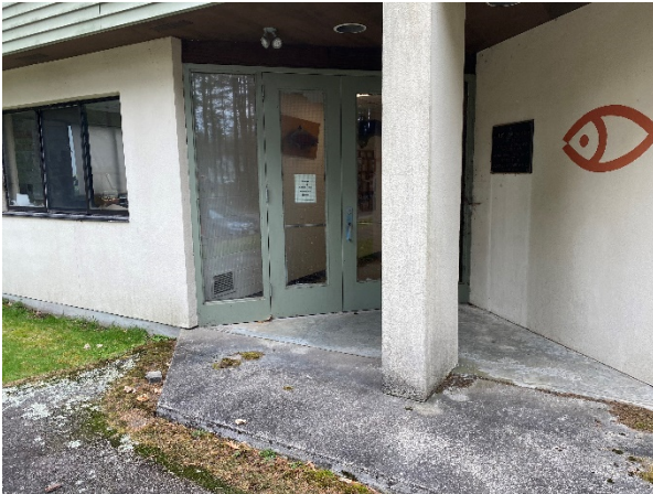
Figure 5-8: Main Entrance Doors
