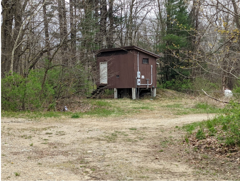
Figure 4-5: Old River Well (No. 3) Structure
