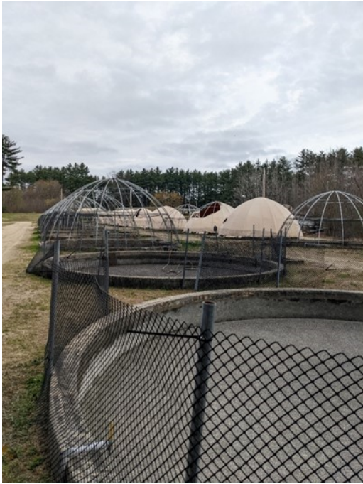
Figure 5-26: View of Lower Circular Tank Area
