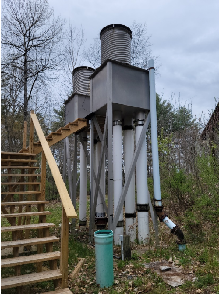
Figure 4-8: Aeration/Degassing Headbox
