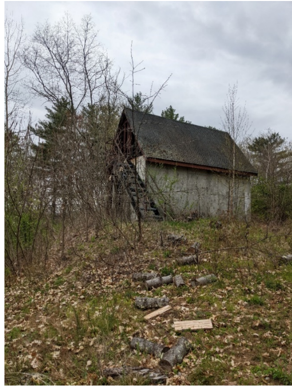
Figure 4-7: Older Aspiration System Building (no longer in use)
