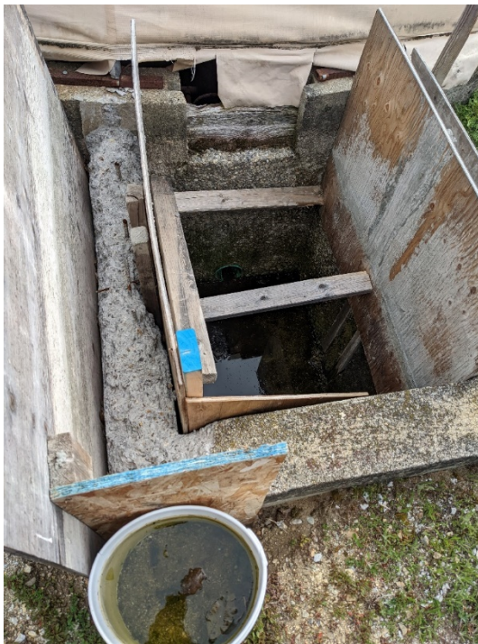
Figure 5-32: In-Process Concrete Repairs of Circular Tank Outlet Box
