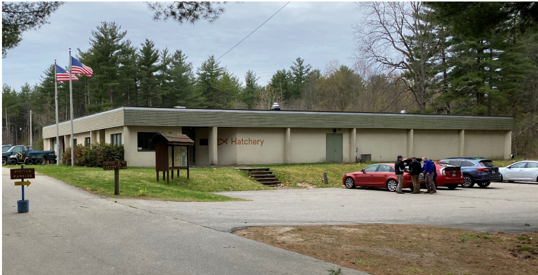
Figure 5-1: Hatch House (View of Front Entrance)
