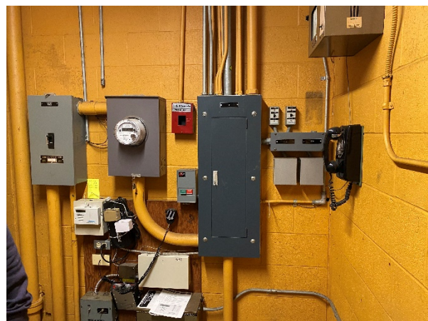
Figure 5-24: Electrical Room East Wall
