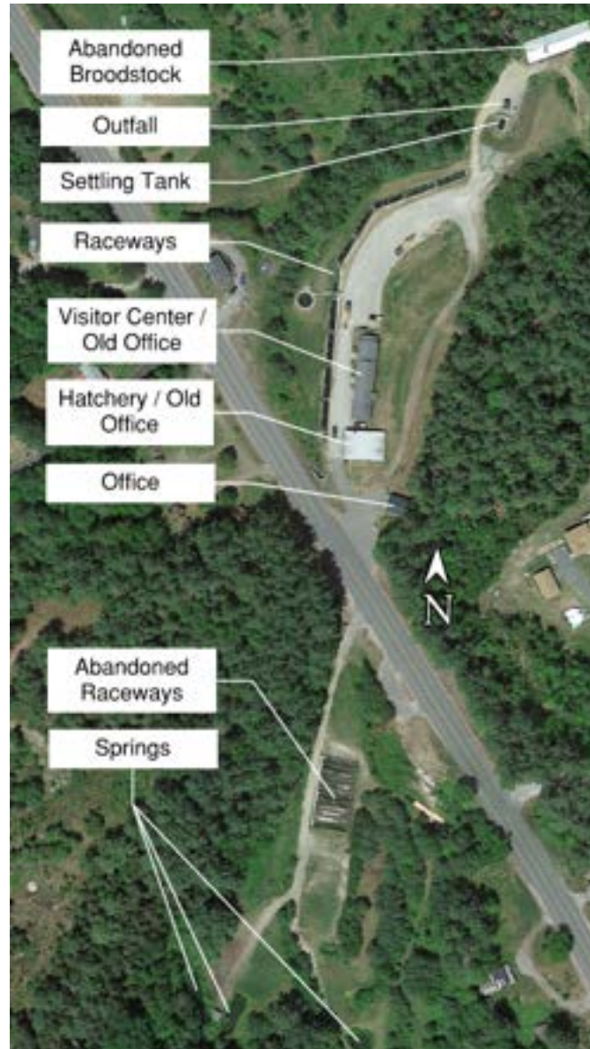
Figure 2-6: Twin Mountain State Fish Hatchery Aerial Image.
