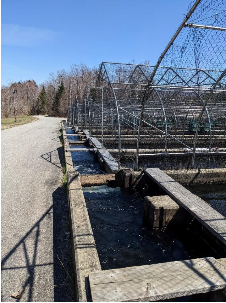
Figure 5-15: West Branch Raceways
