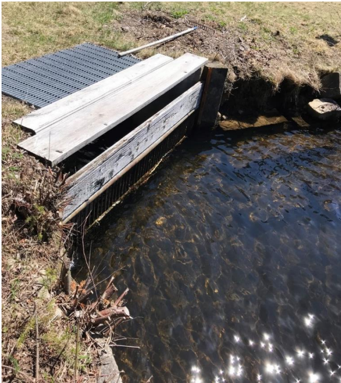
Figure 4-11: Diversion Pond Outlet Structure to Raceways
