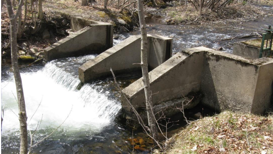
Figure 4-8: Third Brook Diversion and Intake Structure
