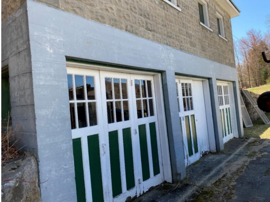
Figure 6-5: Pipe Shop Lower Level Carriage Style Garage Doors
