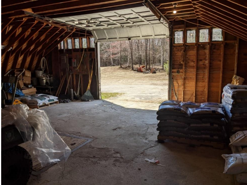
Figure 6-2: Feed Storage Building – Upper Floor Interior
