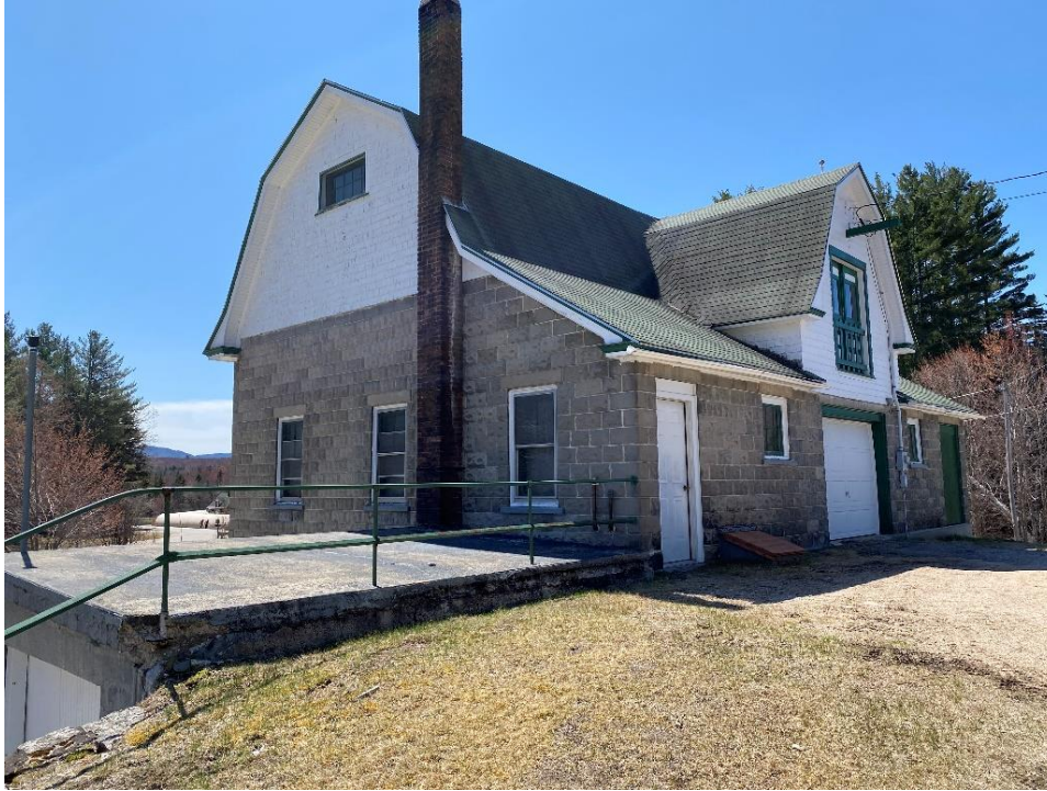
Figure 6-11: Carpenter's Shop North and West Facades
