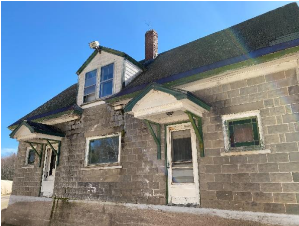
Figure 6-24: Q2 Front Facade
