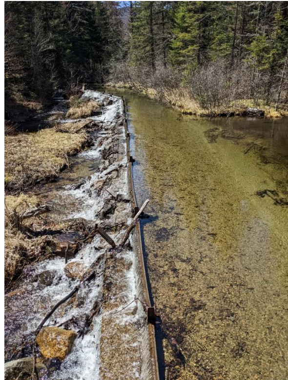
Figure 4-10: West Branch Diversion Dam
