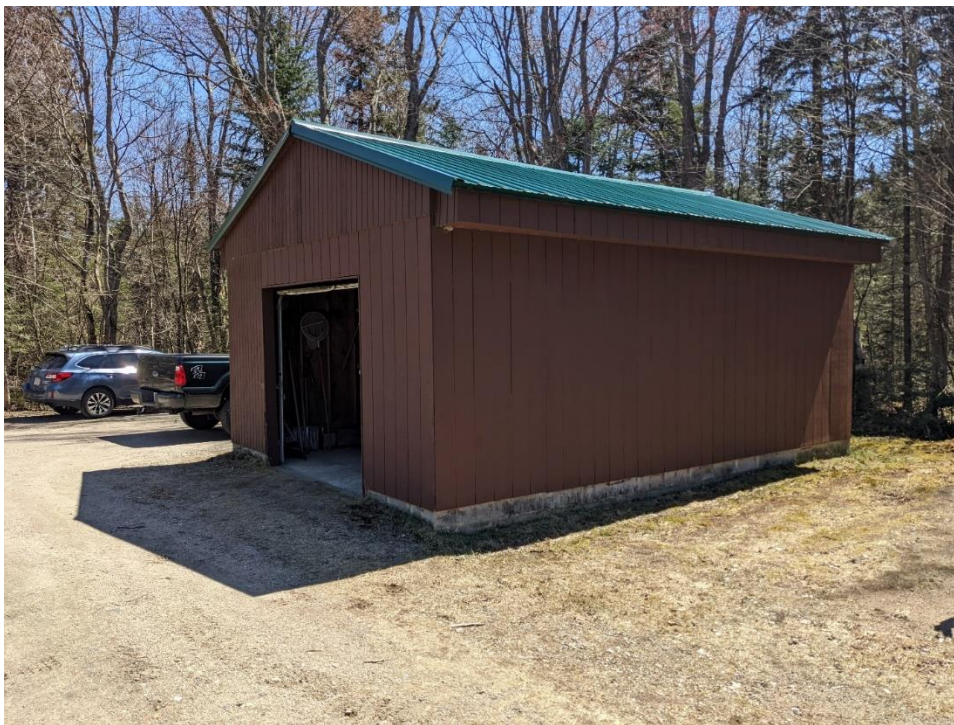
Figure 6-18: Upper Canal Garage
