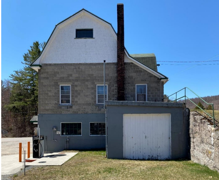
Figure 6-14: Carpenter's Shop Storage Garage and Gas Pump
