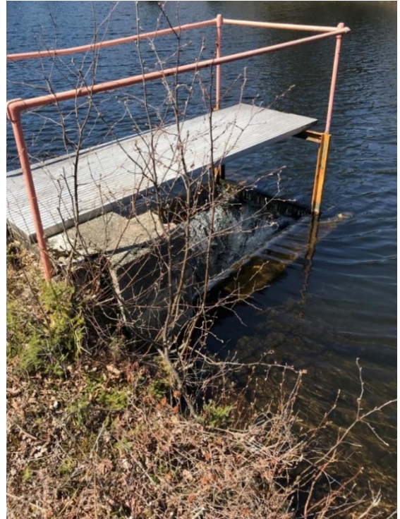
Figure 4-13: Diversion Pond Outlet Structure to River
