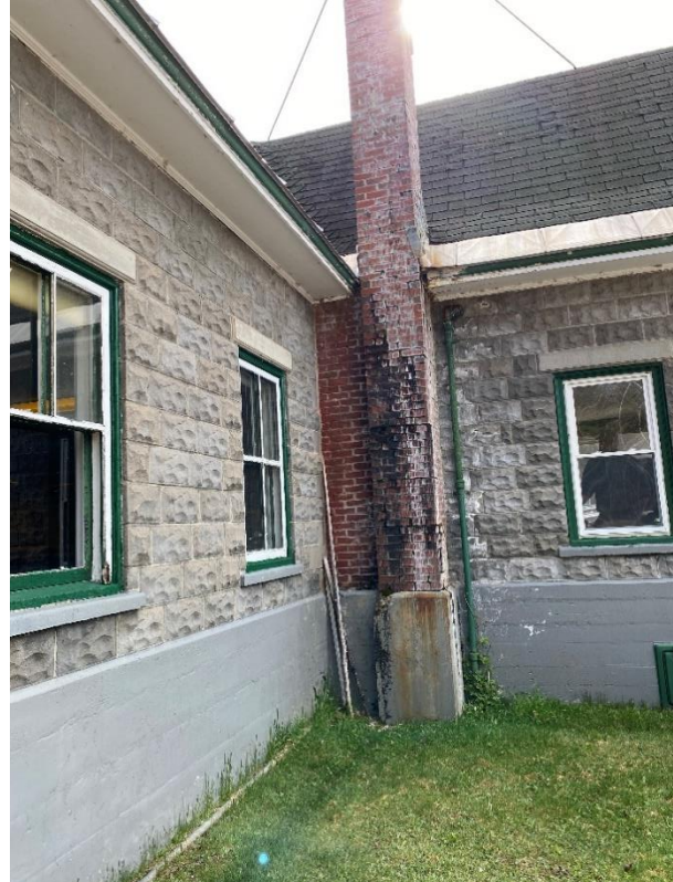
Figure 5-4: Main Entrance Chimney
