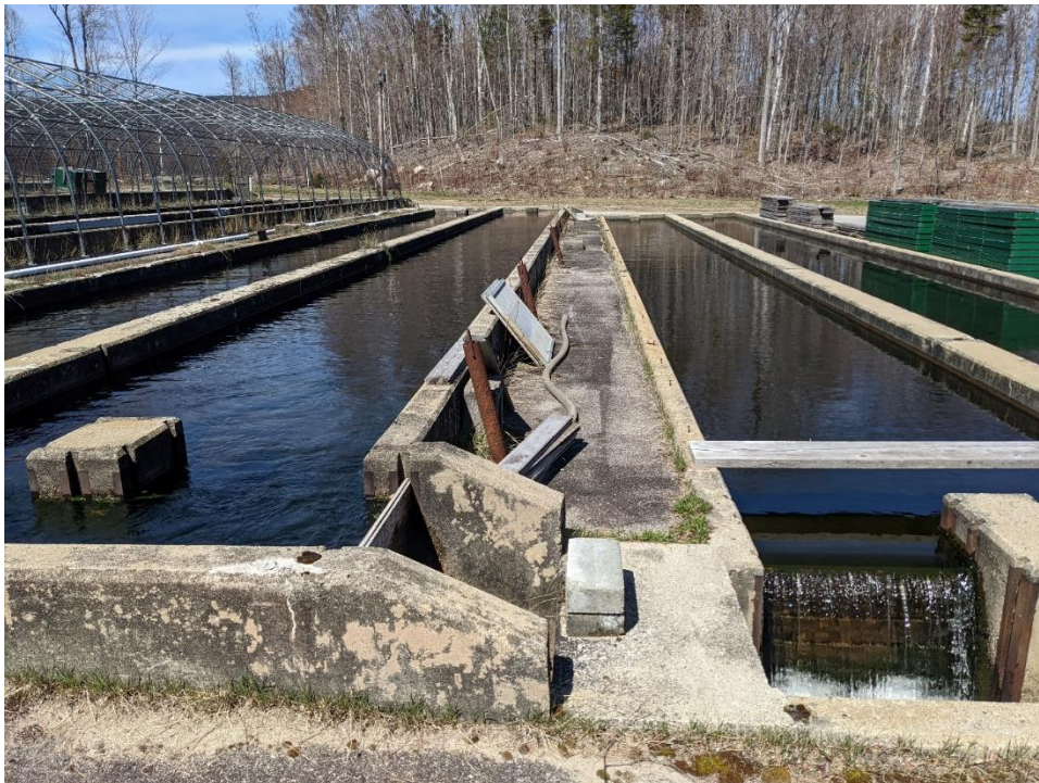
Figure 5-17: West Branch Raceways Settling Channel
