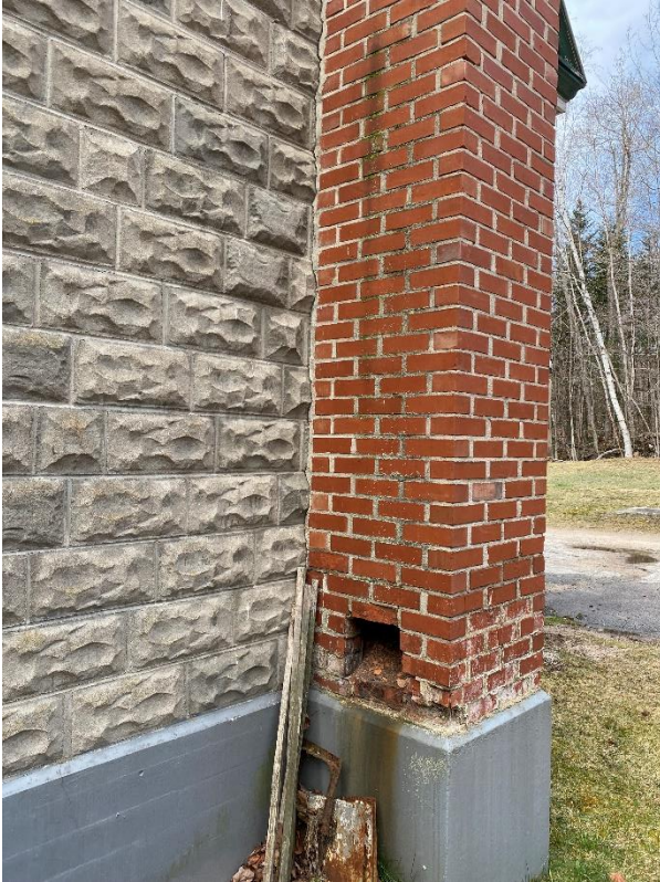
Figure 5-3: Boiler Room Chimney
