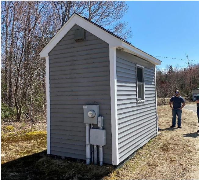
Figure 5-18: West Branch Sampling Shed
