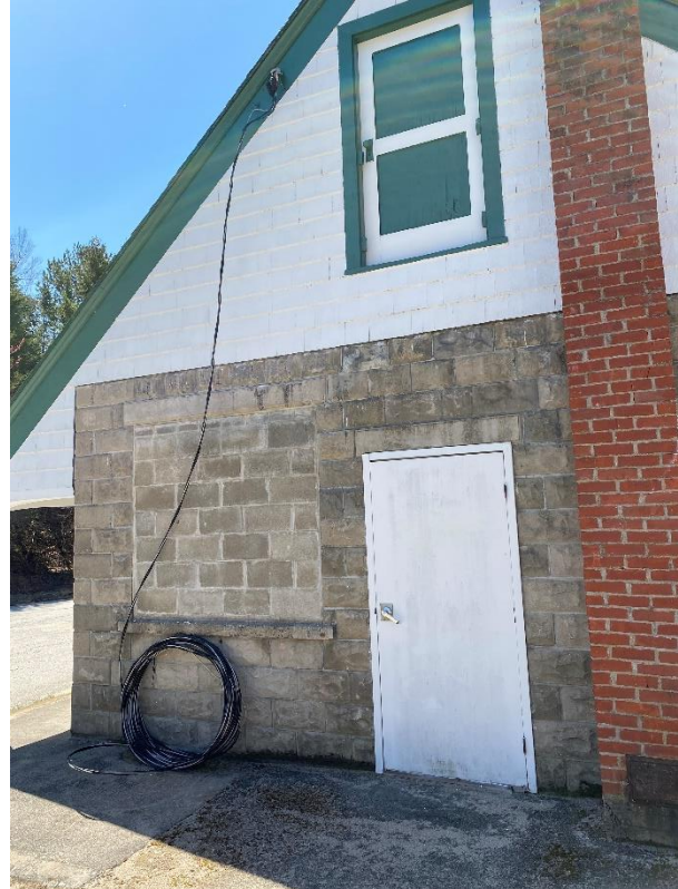
Figure 6-23: Visitor's Center Egress Door and Attic Access
