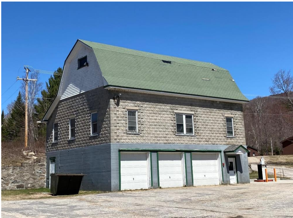
Figure 6-10: Carpenter's Shop South and East Facades
