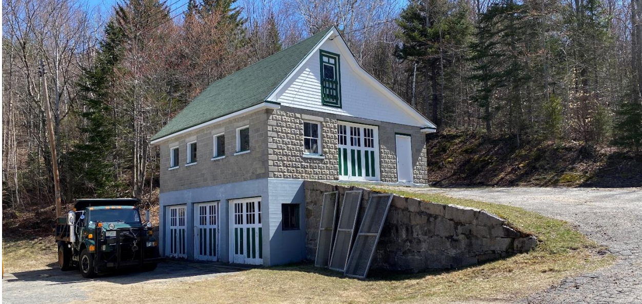
Figure 6-4: Pipe Shop Overall View
