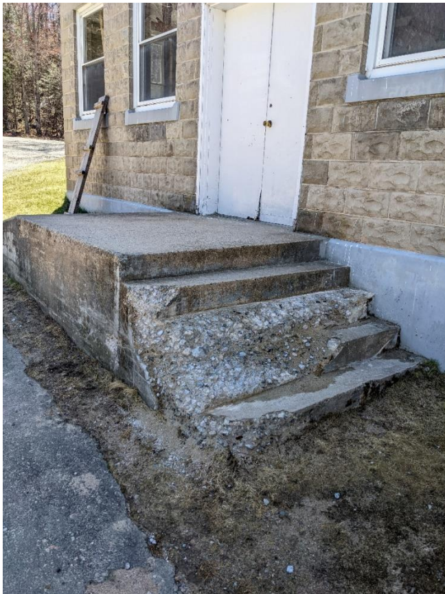
Figure 6-3: Feed Storage Building – Front Steps
