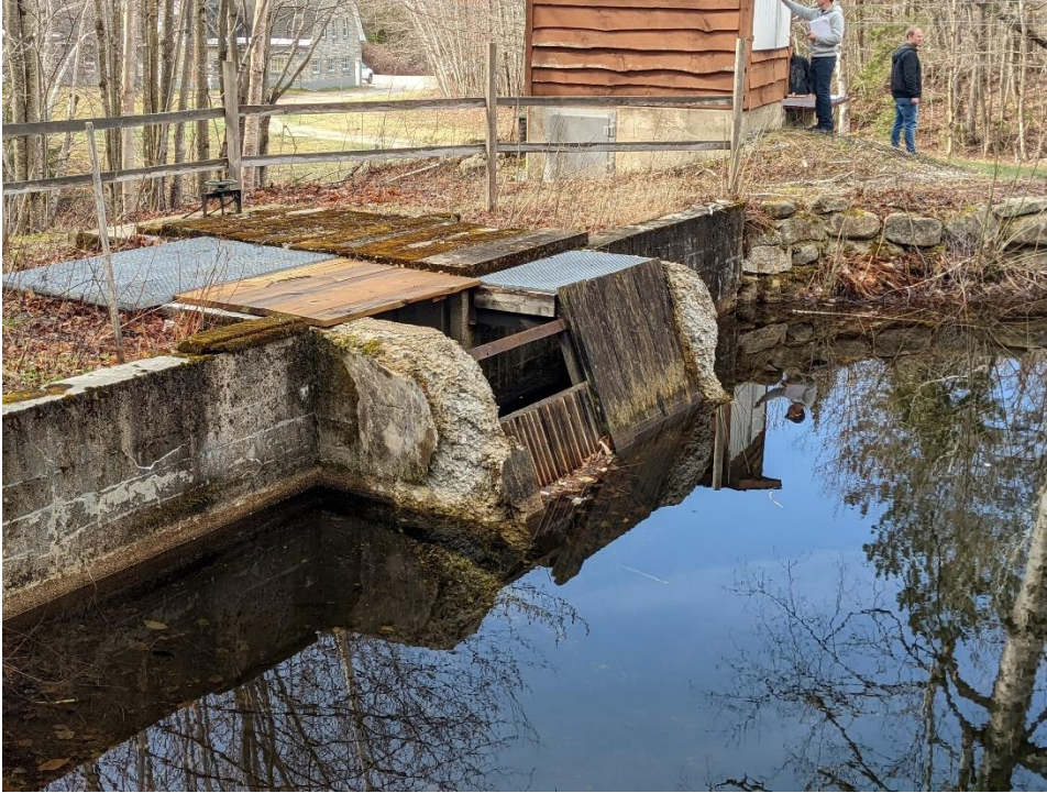
Figure 4-3: Salmon Pond Outlet and Distribution Box
